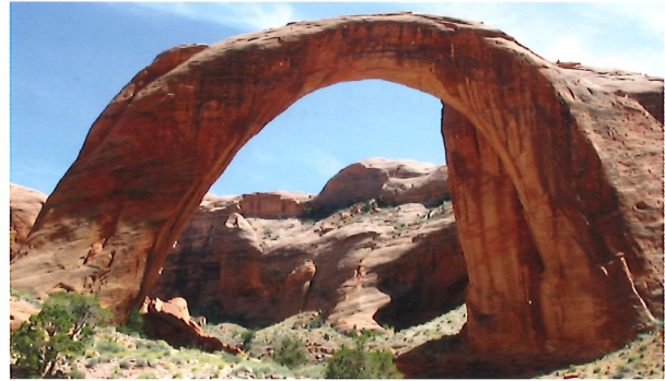
Bild 9.1: Sandstein-Bogenbrücke Rainbow Bridge National Monument in Utah, USA (Foto: National Park Service)
